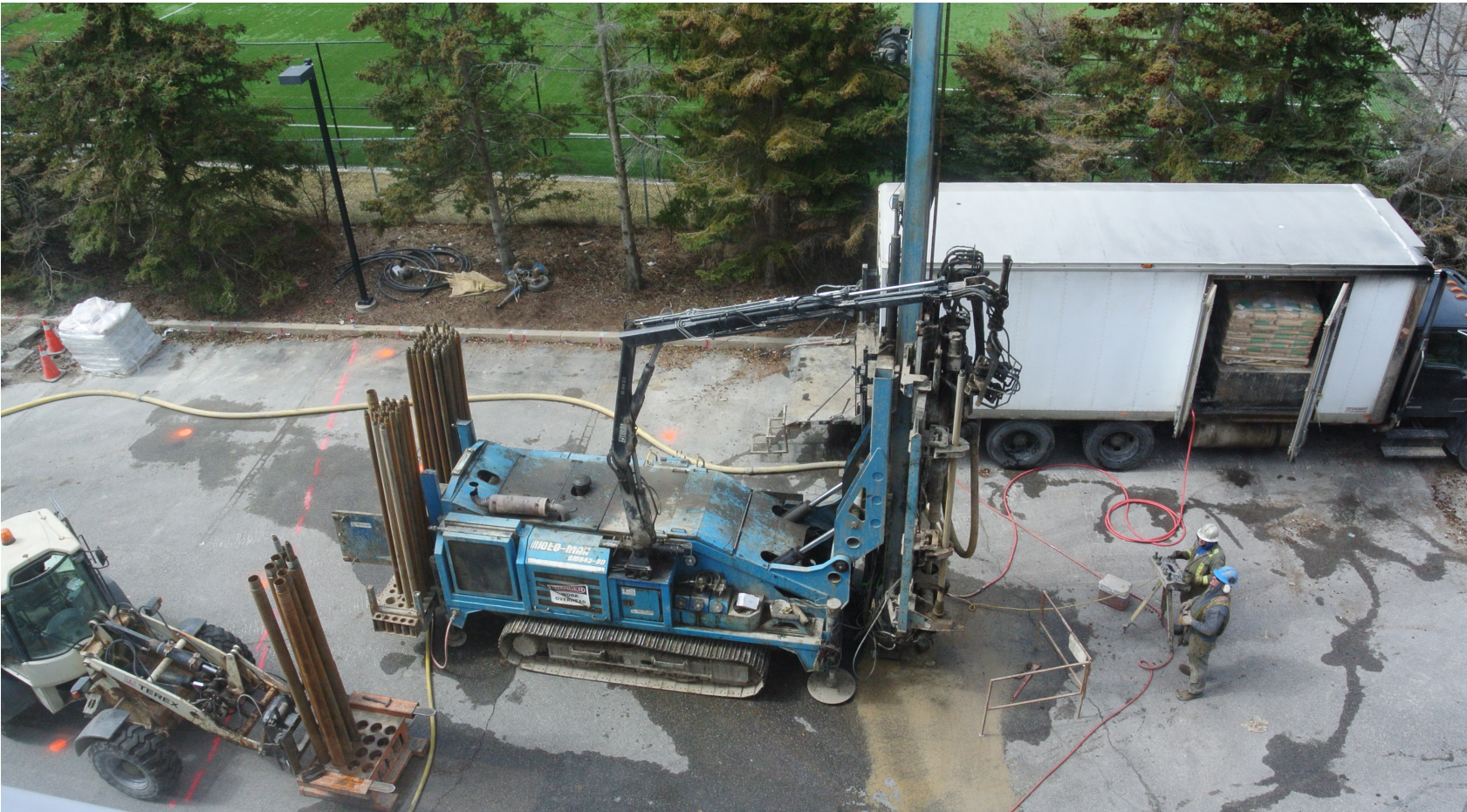
Figure 13: Geo-thermal wells are drilled into the west parking lot at 111 Moatfield
